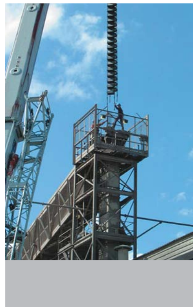
Figure 17: quick and simple assembly of a HEKO endless chain strand
