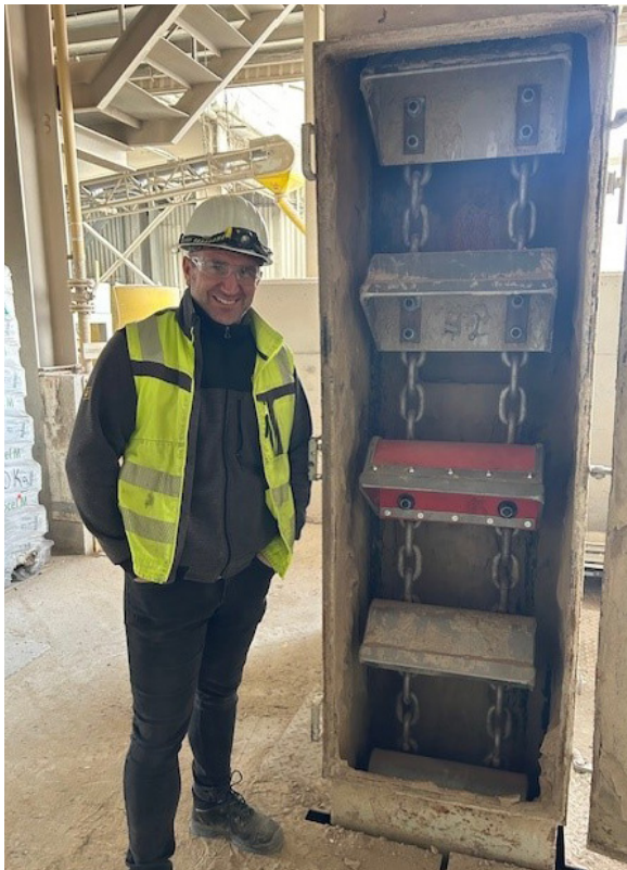
Figure 7. B. Bergmoser in front of the new equipped sand and gravel bucket elevator at the Spenner cement plant in Erwitte.
